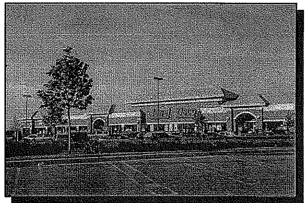
Encouraged example of big box architectural treatment
